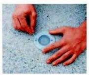
Step 5 Insert AQUALED<sup>®</sup> into the outer casing and screw the fixing ring to this casing.
