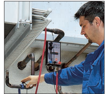
Measuring subcooling using an attached pipe wrap probe
