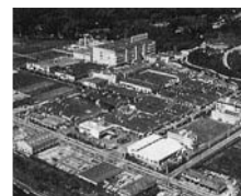
KYOCERA Kagoshima Sendai Plant
