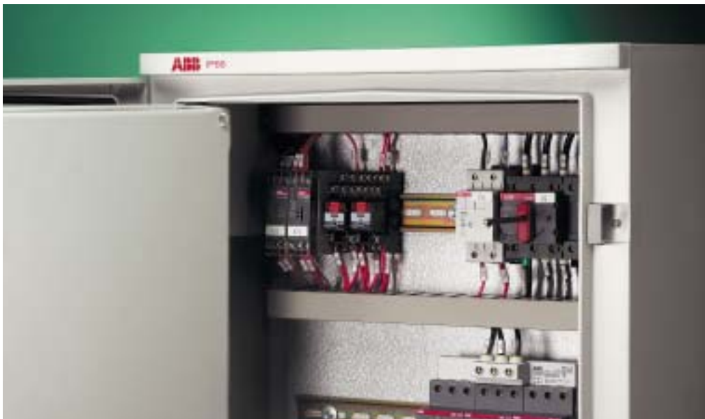
Application of the inner door guarantees IP40 degree of protection when the switchboard door is open.
